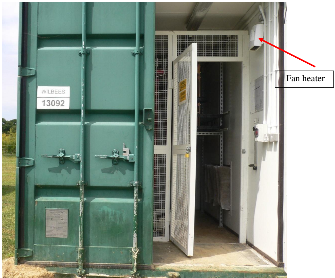
Figure 7 : HV switchgear zone showing location of the heater
